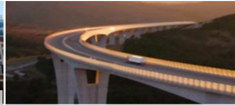
KRINKAL BRIDGE - SLOVENIA
